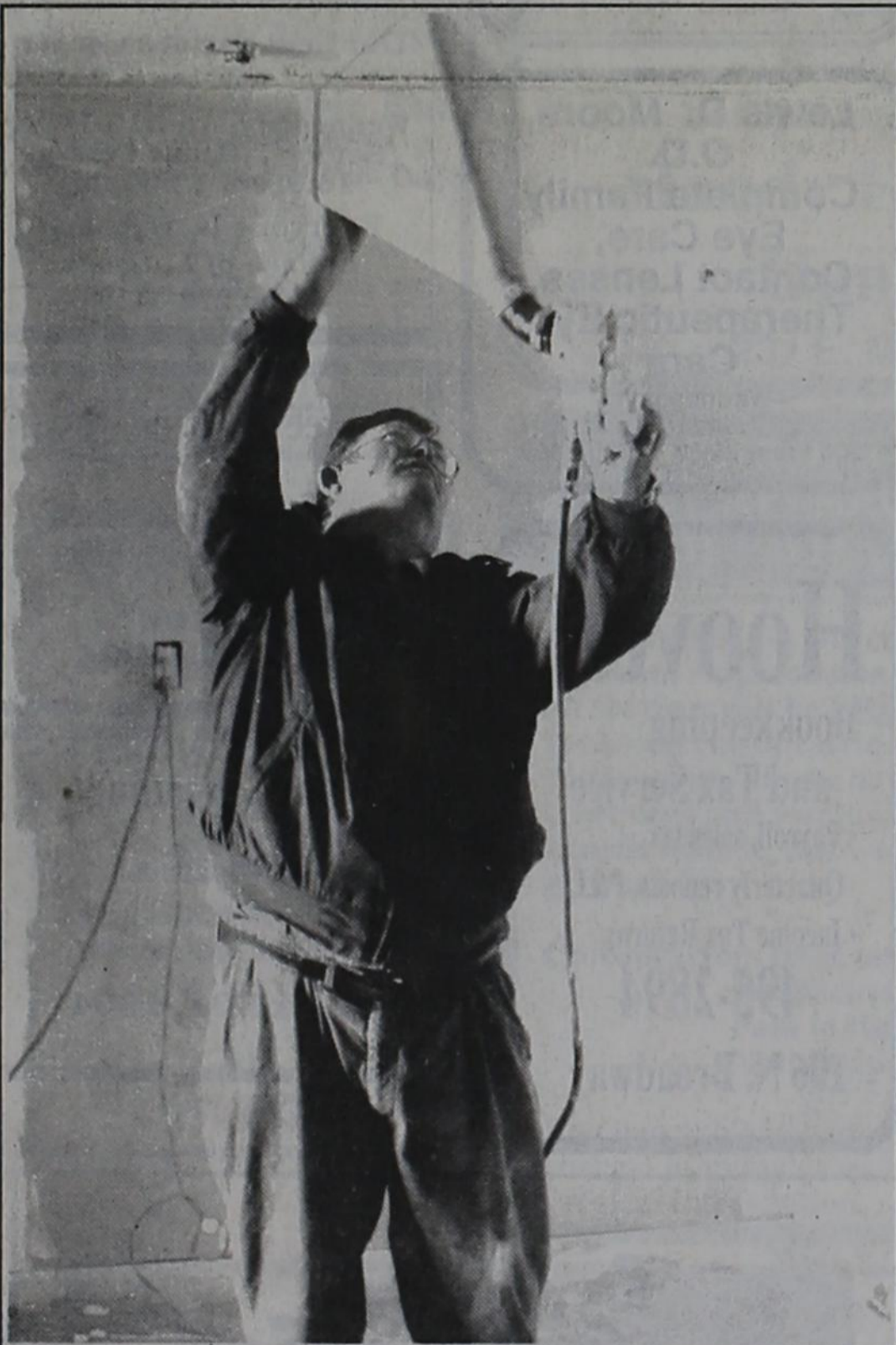
BOB CHENNAULT sprays an acoustic ceiling in his booth at the old Postex Mill
