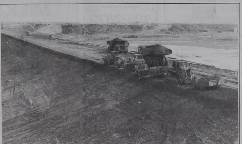
tenants of the land. The land was part agreement as the original lease that ACLOSER view of the dam shows some of the heavy equipment that is being used to haul in the more than six and a half million cubic yard of earth used in the construction of the project. (Photo by John Cordsen)
