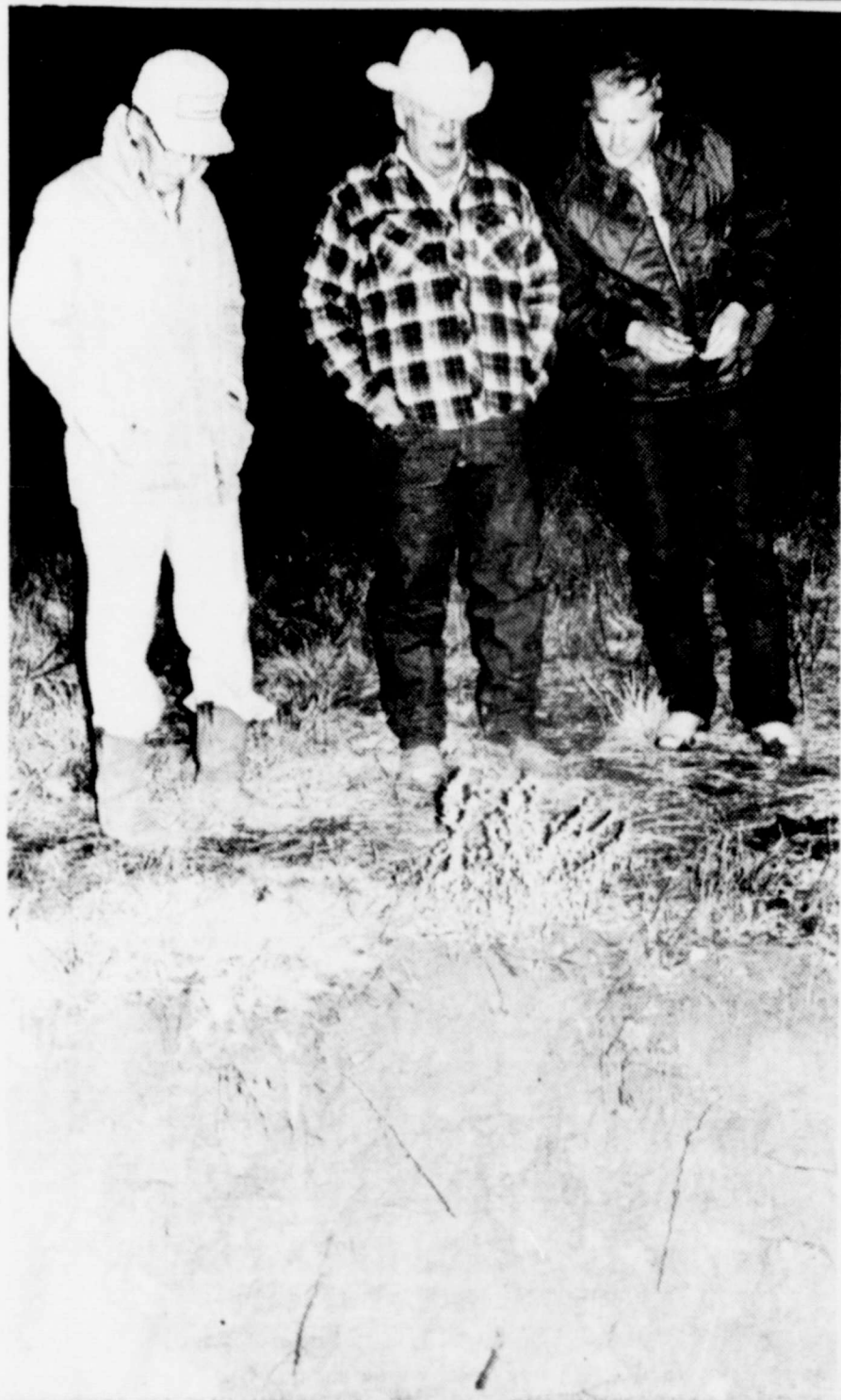
Merkel mayor Kent Satterwhite, [left], city manager J. A. Sadler [center] and a member of the Tye Volunteer Fire Department look at the break in the city's main water line. The leak was discovered by the city's crew at 3 p.m. Sunday and was quickly repaired overnight. A replacement collar was welded and then cemented into place early Monday morning. Water service was restored in most parts of the city by 8 a.m. Staff photo
