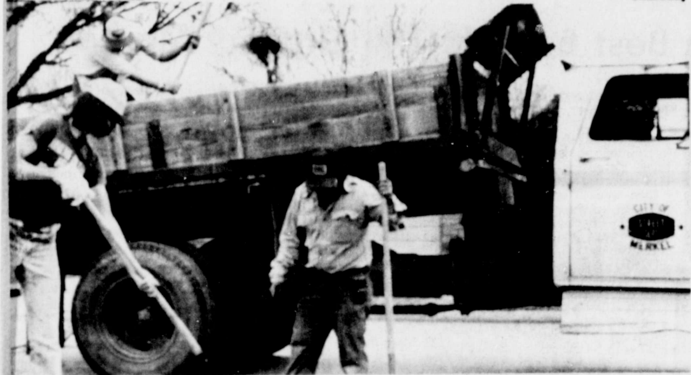
Danny Frazier, Calvin Boone and Ray De la Cruz have started filling in the potholes left by rough winter conditions here. The West Central Texas Council of Governments is still looking for three
