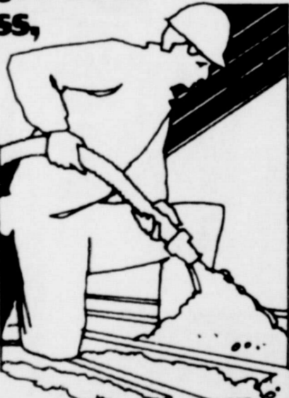
ThermoCon loose-fill insulation is blown in to attics with no insulation - and as a topping over present insulation.
