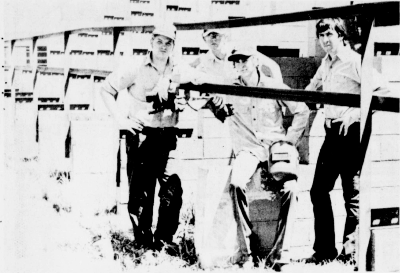
REPAIR STANDS --Members of the Trent High School Agriculture Mechanics class are busy this week getting the football stadium seats rebuilt in time for Friday's opening contest. The students aligned and welded railings and placed
