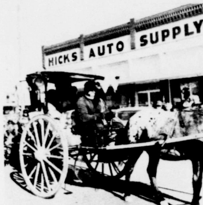
TAYLOR ELECTRIC CO-OP first place
