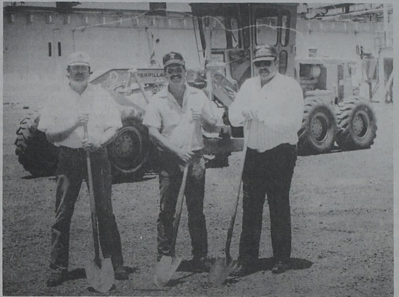
READY TO GO.... A ground-breaking was held at Friona's Excel plant last week for the $11 million expansion project at the plant. From the left are Guy Hunter, project manager; Randy Highsmith, construction engineer; and Jack Messer, contractor. Not present was Don Determan, Excel's plant engineer. On-site work has begun, and actual construction is expected to get underway on the project in the next 30 days.
