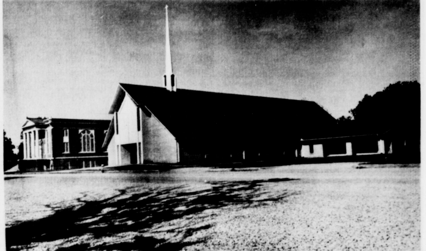
NEW SANCTUARY of the First Baptist Church. Dedication services are to be this Sunday at 11 a.m. Rev. Kenneth Jones is pastor of the church. Pictured in the background is the old building.
