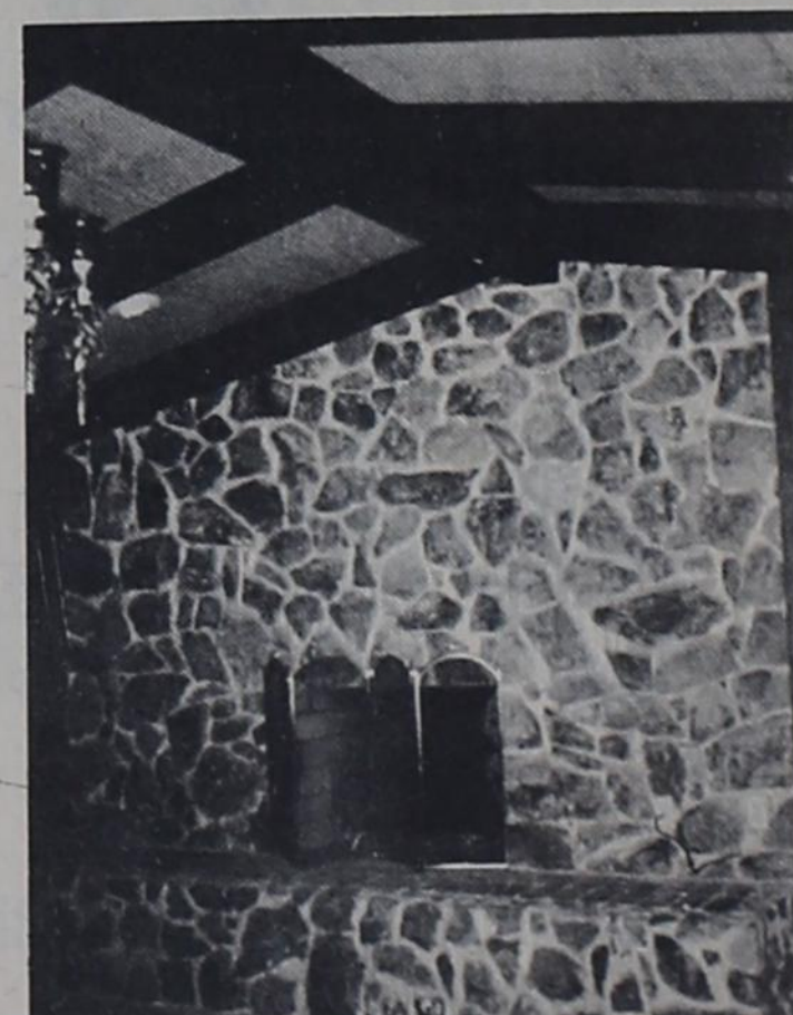
SHOWN IS the beautiful rock fireplace in the new home of Mr. and Mrs. Billy Johnson, which was built by Nowlin, Embry and Smyer.
