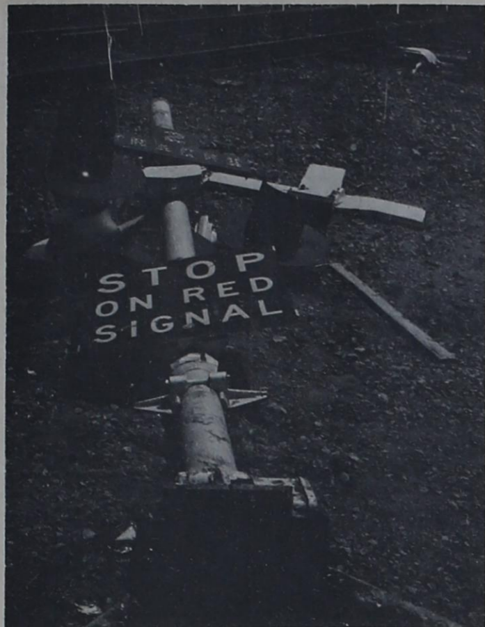
COLLISION --- The signal light on the north side of Santa Fe tracks at the Third Street crossing was knocked from its moorings Tuesday afternoon when struck by a pickup. Driver was not injured. A new signal was installed that same afternoon within two hours.
