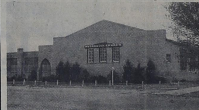
Oklahoma Lane Methodist Church
