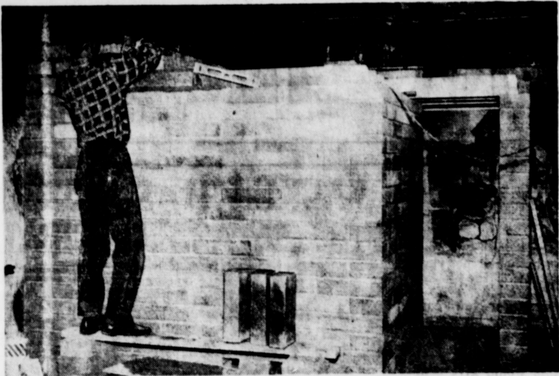
FAMILY FALLOUT shelter constructed in the basement of the Orval M. Conner residence in Battle Creek, Mich., is typical of some 100 built or planned in the nation of either the basement shelter type or the outdoor above or below-ground design. The Office of Civil and Defense Mobilization is building the various shelters for research and demonstration purposes. Group and community shelters are also among 150 projects now under way or being negotiated throughout the nation for construction in new and existing public and private buildings, in parks, and similar sites. (OCDM Photo)
