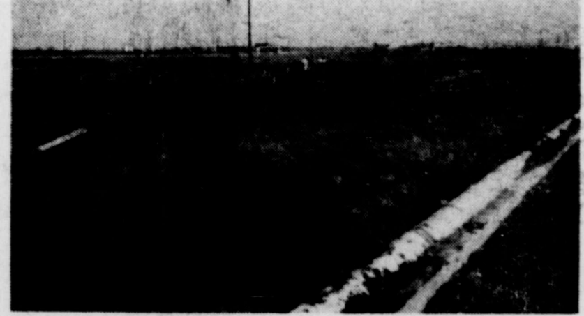
Housing Site —Curbing is in and work underway on Merkel's $227,700 low rent housing project in the northeast part of town. Construction is expected to be completed in August.
