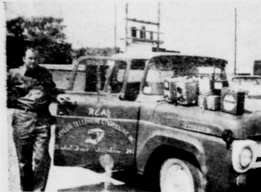
TEST EQUIPMENT — Bob Huckaby is shown with truck that carries testing equipment for Taylor Telephone Cooperative, Inc. Huckaby is inside superintendent for the phone co-op.
