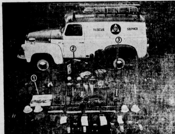
eral Civil Defense Administration for Federal equipment; (2) portable inhalator, and (3) port-matching funds, has an amazing array of equipable one-kilowatt generator. Four-wheel-drive matching funds, has an amazing array of equip-ment for its four-man crew. Included are: (1) truck can traverse rough terrain. (FCDA Photo)
