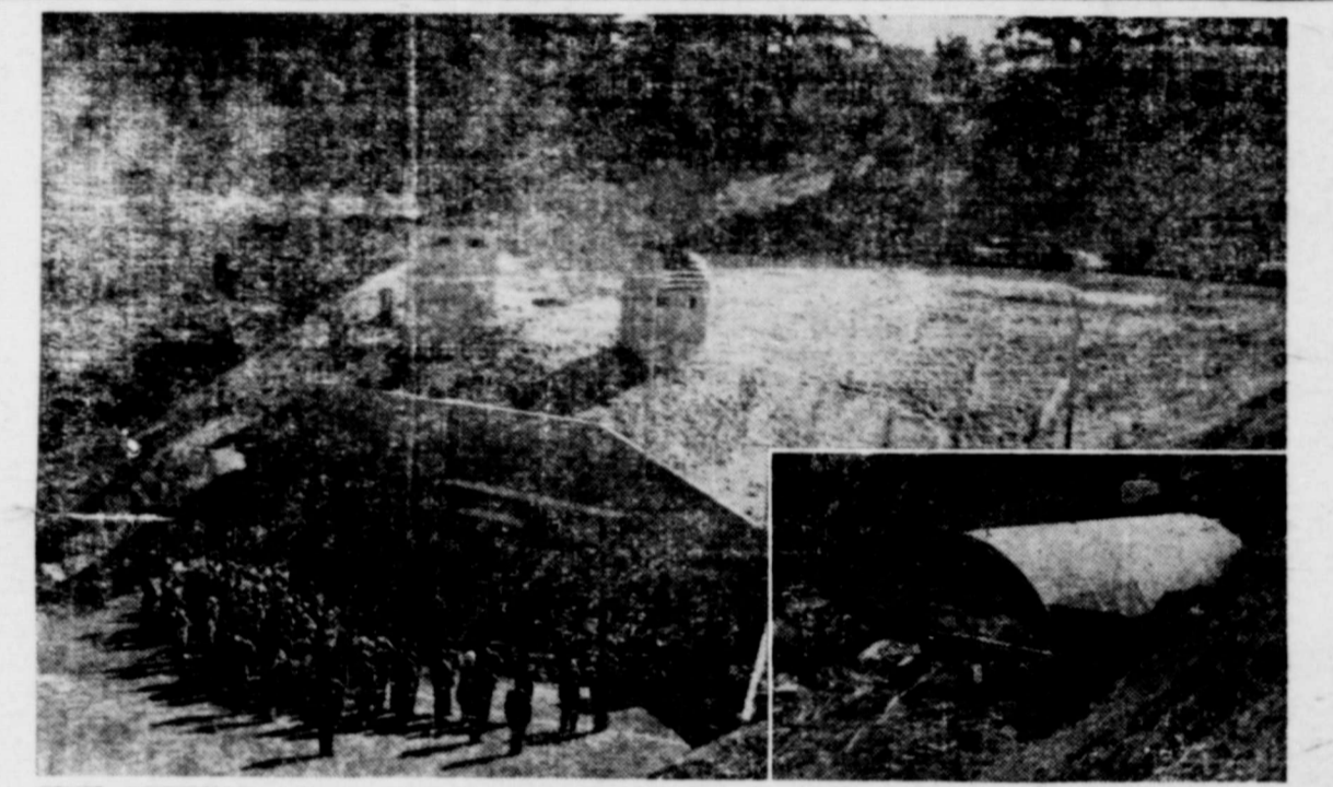
CIVIL DEFENSE underground control center for Portland, Ore., is dedicated at the site on the outskirts of the city. Center is equipped with heavy electric entrance doors with photo-electric alarm and closed-circuit TV control of personnel entering, air locks and radiological decontamination facilities, electric generators, a private radio station, air filter and ventilation system, telephone, press and Comelrad facilities, and space for civil defense and other emergency offices. In addition, the $667,000 structure includes space for weather and radiological specialists, and living facilities. Inset shows arch construction of control center. (City of Portland and Oregon Civil Defense Photos)
