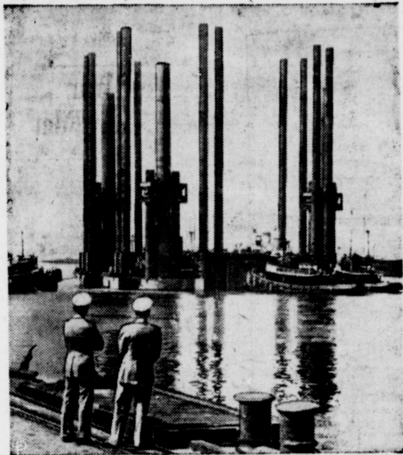
TWO NAVAL OFFICERS watch as the 6,000-ton Texas tower radar station, surrounded by a fleet of tugs, leaves Boston Harbor on its way to sea. The huge platform, which will resemble a three-legged stool, will be set up as an island about 110 miles east of Cape Cod.
