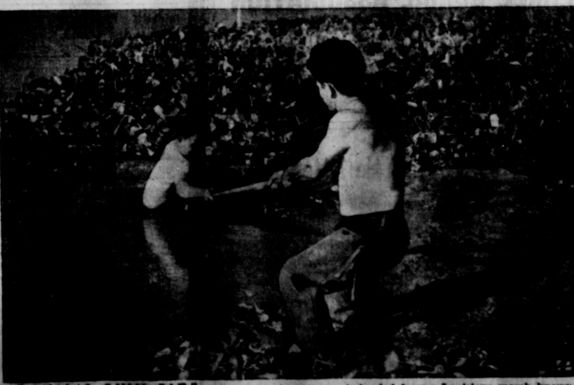
DEVIL'S OWN SITE — A surveyor's crewman is hauled from a Louisiana marsh known as Garden Island Bay where a sulphur company will mine 500,000 tons of brimstone yearly.
