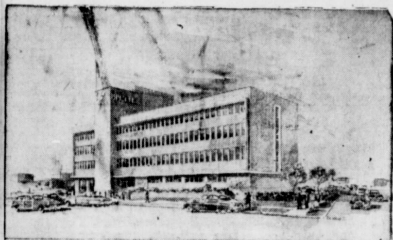
New office building for Humble Oil & Refining Company's West Texas Division headquarters in Midland.
