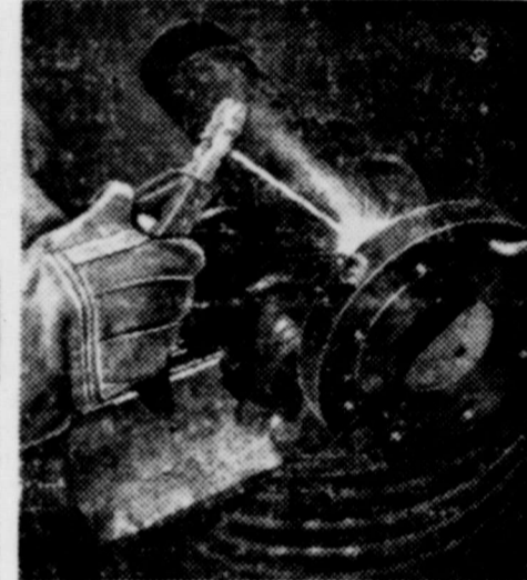
THEY WELD PIPE
