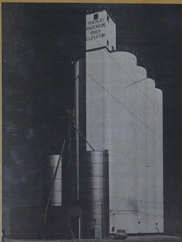
SHERLEY-ANDERSON RHEA ELEVATOR JOE ALLEN
