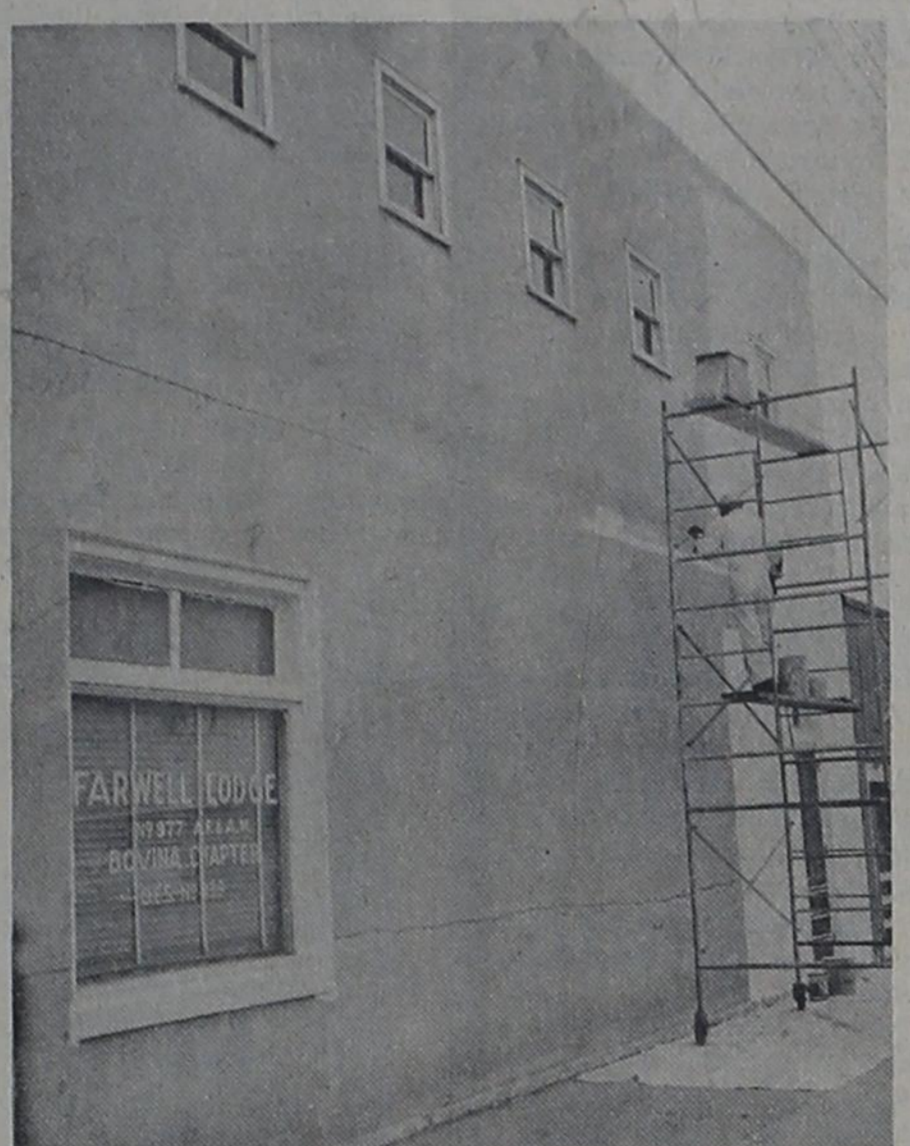
NEW PAINT --Masonic Lodge Hall here is receiving a face-lifting this week. A new coat of white paint is being applied to the two-story building by Contractor Howard Griffin. Woodwork on the stucco building will be painted black. Griffith, who began the job Monday, estimated that it would take about a week.
