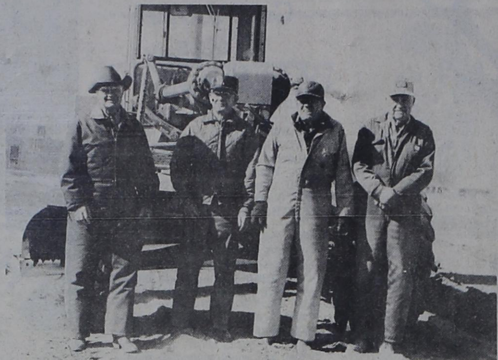
NEW SENIOR CITIZENS SITE .... being cleared off and leveled. The new center will be located at the corner of First and North Streets, just east of the old Bovina Supermarket.
