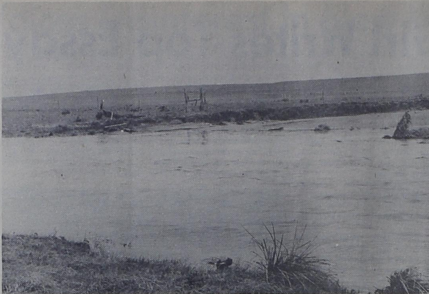
COUNTY RESIDENTS were reminded last week of the importance of the Running Water Draw watershed project when the flood-like rains sent the draw on a rampage once again. This picture was taken south of Friona. (SCS photo)
