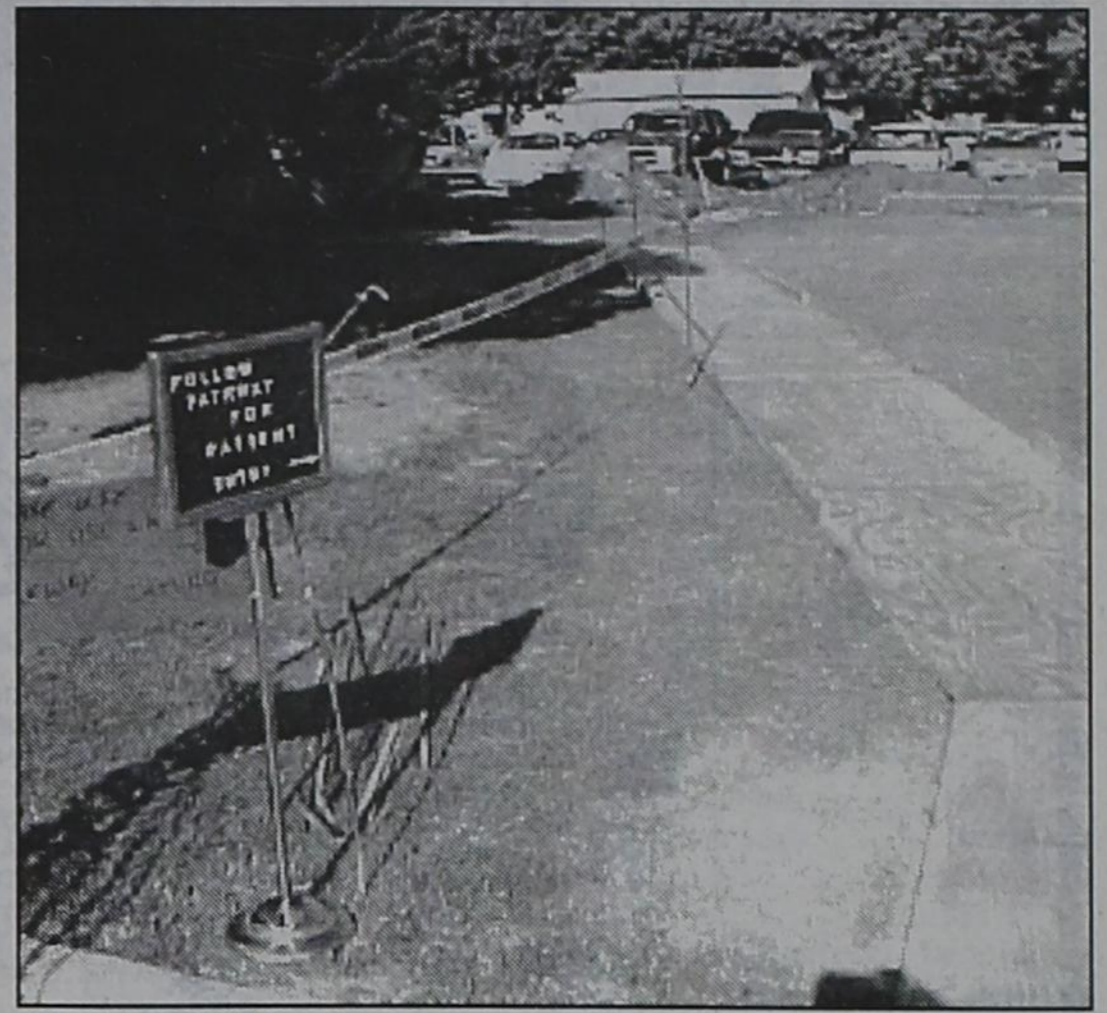
NEW ENTRANCE AT PCCH.....Due to construction, a temporary entrance has been necessary. The plywood sidewalk, above, leads to an entrance at the north end of the hospital.
