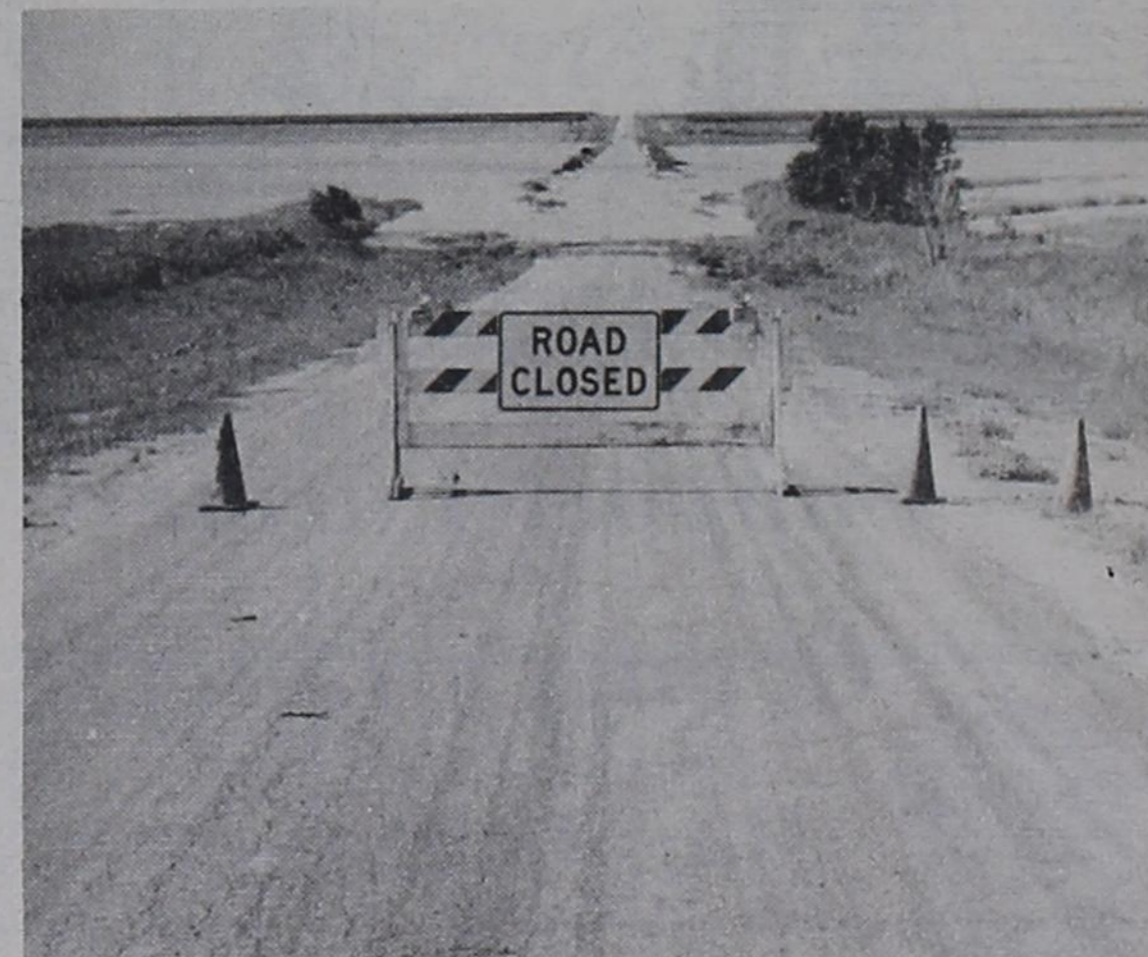
ROAD CLOSED TO TRAFFIC.... But what about boats? Shown is Twin Lakes as they covered the roadway with water. Recent rains have filled up the lake to overflowing, and sources say this is the first time in several years that the lakes have been over the roadway.
