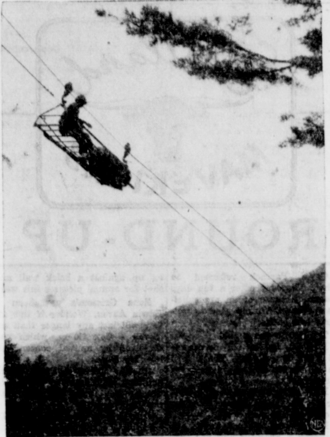
THE LINE IS BUSY—Riding high above the rugged mountain peaks on the Central Front in Korea, a U. S. soldier of the 7th Division uses a aerial tramway that hauls supplies to UN front-line troops. The high-wire transport system, rigged by U. S. engineers, hauls men and supplies with equal ease. (NEA-Acme photo by Staff Photographer Jim Healy.)
