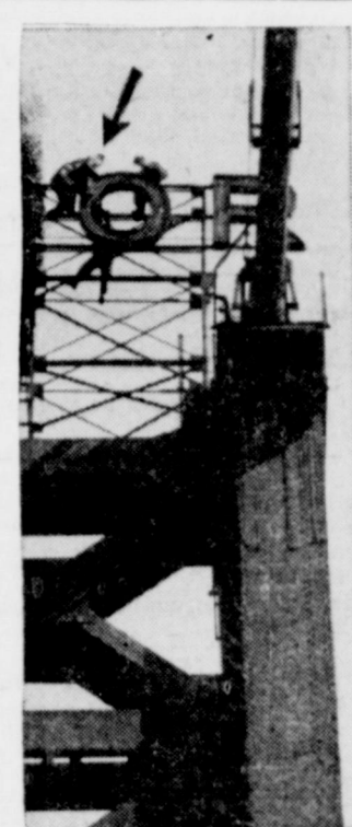
TO THE RESCUE—After a fearful struggle as he sat atop the 386-foot Ambassador bridge, Harry Sandlin (arrow), 24, was finally subdued by maintenance men and brought down from his lofty perch. It took over one hour to get Sandlin, an unemployed factory worker, down from the bridge which spans the Detroit River. (NEA Telephoto.)
