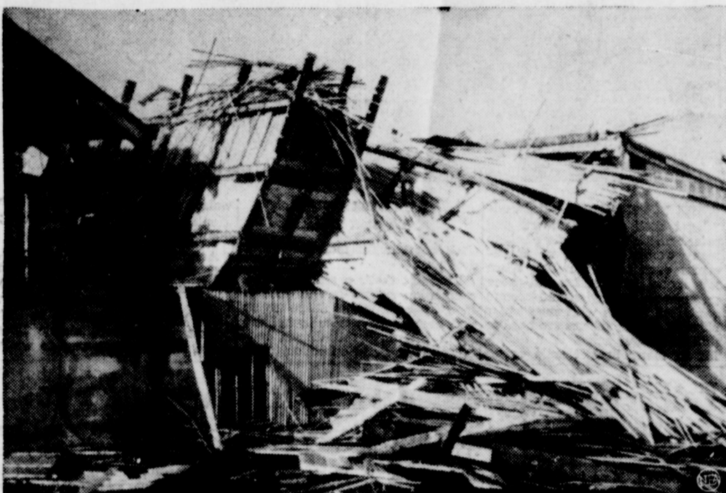
TWISTER HITS OKLAHOMA CITY —When a freakish tornado skipped across Oklahoma City, Okla., it left in its path a series of unusual things. This is a view of a sash and door manufacturing company, showing lumber scattered, a rack of finished doors, left, leaning precariously, but otherwise undamaged. One person was slightly injured. (NEA Telephoto)
