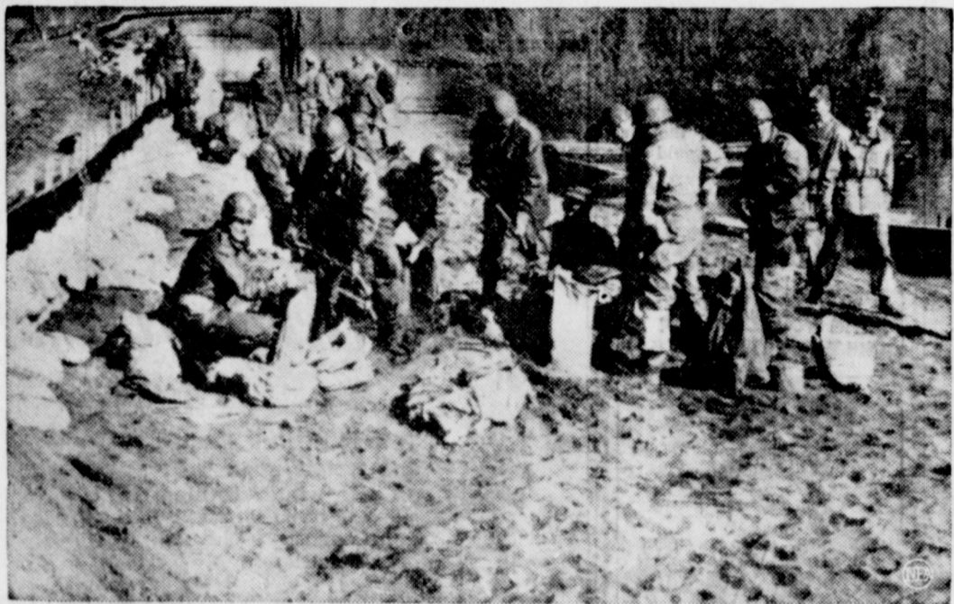
NATIONAL GUARDSMEN SANDBAG RIVER BANK — Wapello, Iowa. National Guardsmen fill sandbags to prevent flood-waters of Mississippi from flooding some 6,000 acres in Louisa County. Flood waters in this area has inundated many thousands of acres of farm lands and caused much industrial damages in the cities. (NEA Telephoto)
