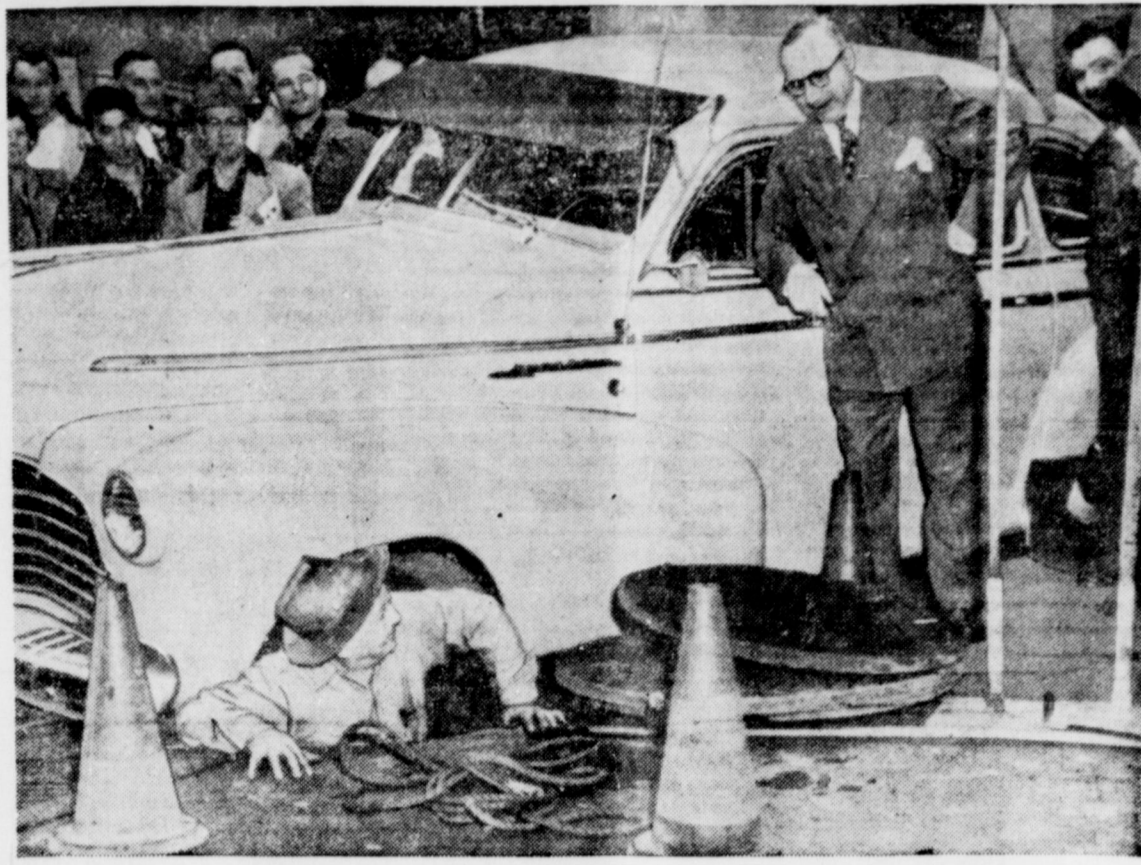
TRAPPED . . . John Ryan, Los Angeles light and power worker, sticks head out of manhole after he was trapped by auto driven by H. R. Marvin (leaning against auto). Marvin was pulling out of alley when car's wheel pushed aside safety screen and dropped into manhole.
