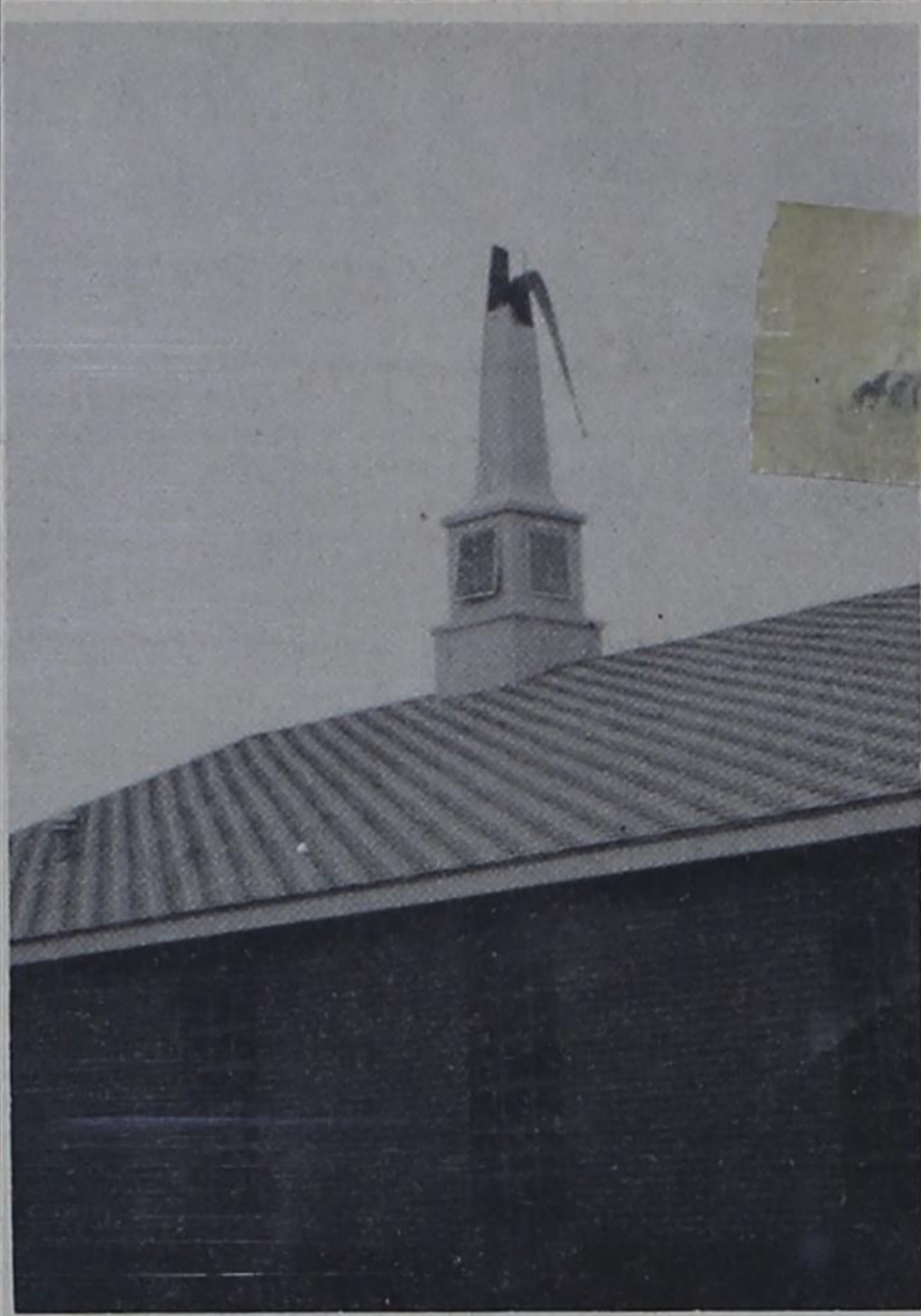
STEEPLE TOPPLES --- Lightning which struck during the noon thunderstorm Thursday apparently hit the steeple of St. Ann's Catholic Church on Third Street causing the upper portion to topple. One bystander said it looked as if "it had been peeled like a banana."
