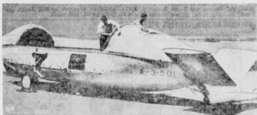
LAST WORD IN AIR-BORNE LIFEBOATS—This new lifeboat, designed to be carried by airplane and dropped by parachute in air-sea rescue operations, would have come in handy during the search for the B-29 that crashed near Bermuda recently. Largest and most completely equipped craft of its kind, the A-3 is nearly 30 feet long and weighs a ton and a half. It has a four-cylinder motor and carries fuel enough to cruise 500 miles. It stocks food and clothing for 15.
