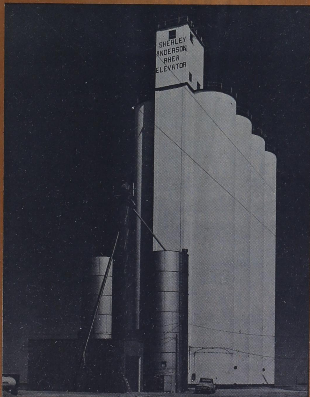
SHERLEY-ANDERSON RHEA ELEVATOR
