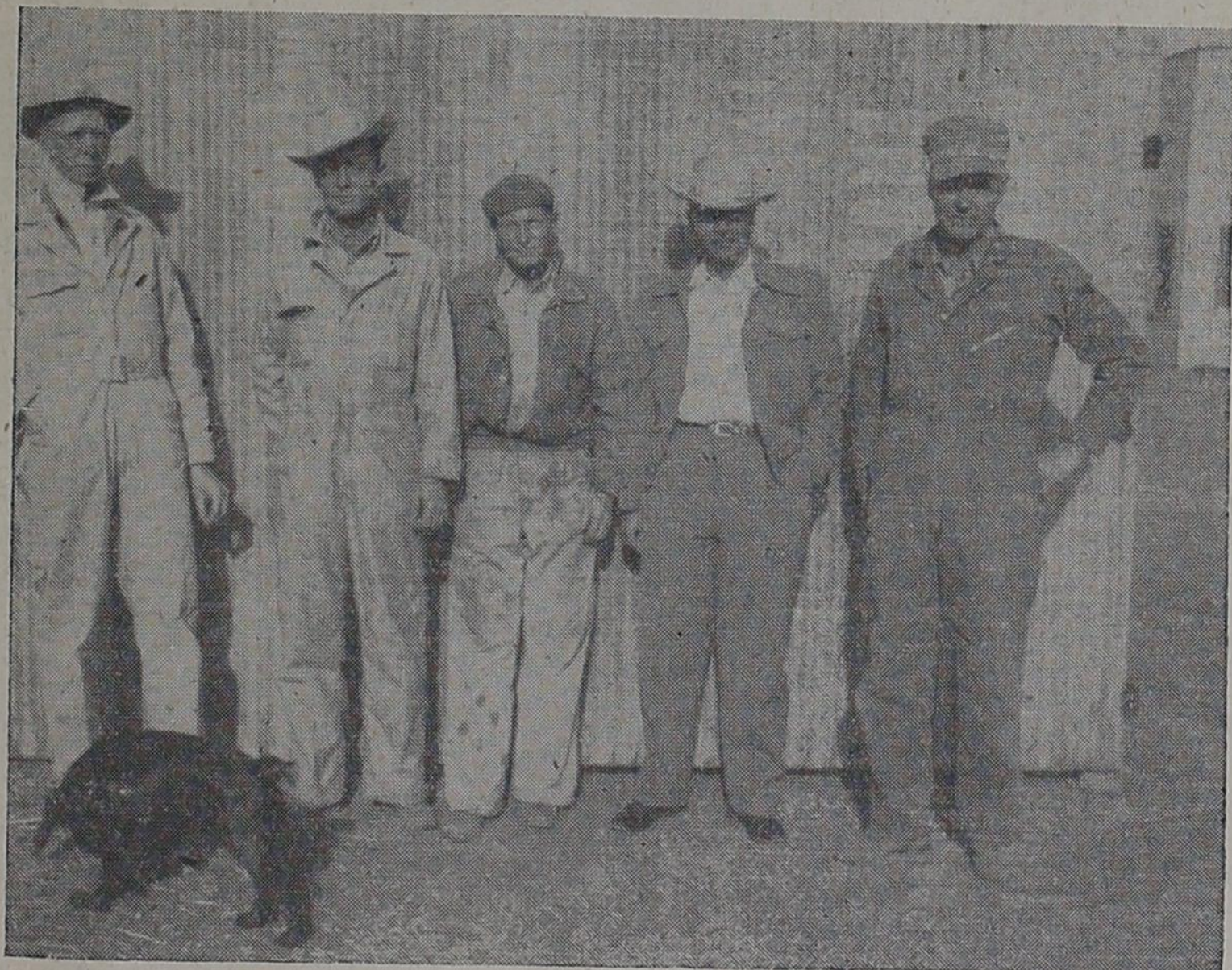
Yes, we are ready to hook your house onto the sewer. Pictured left to right: Hubert Ellison, ditching service; Alva Hudson, plumbing; Odis White, plumbing; Jay Sherrill, manager of Cicero Smith Lumber Company; and Frank Smith, plumbing.
