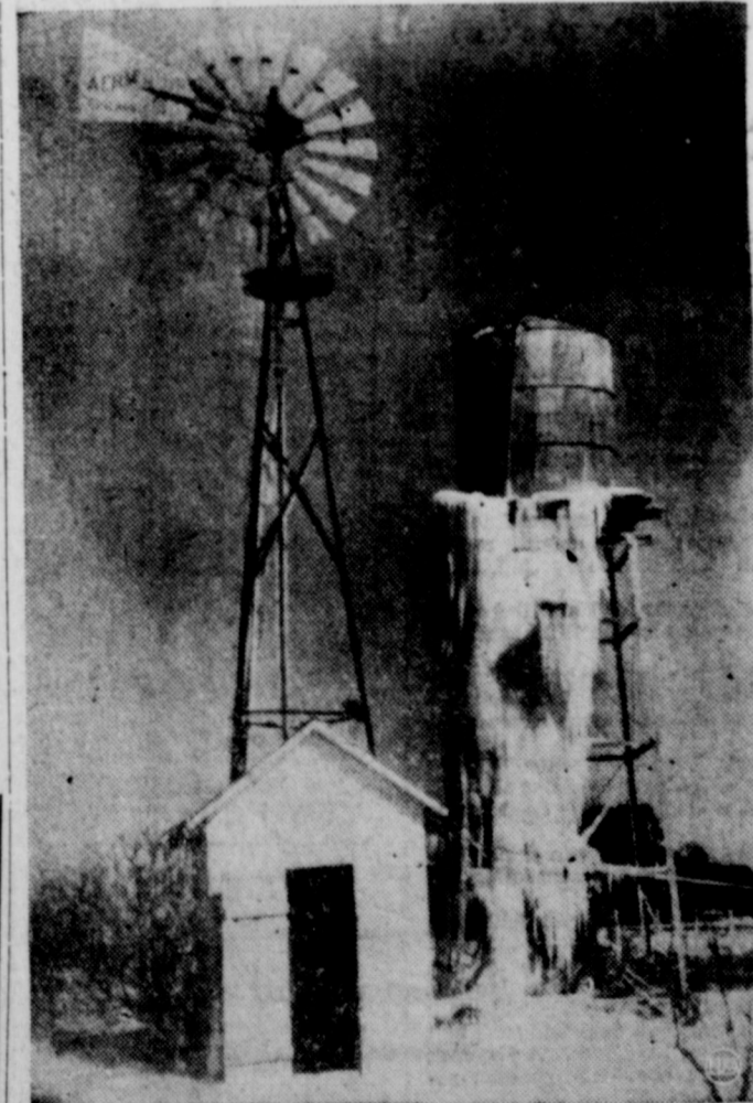
Leaking water from a burst water storage tank in Austin, Texas, froze this 20-foot icicle. Austin, as most of central Texas, was blanketed with over six inches of snow and then was exposed to below zero temperatures. This was coldest the city had witnessed since before the turn of the century. (NEA Telephoto)
