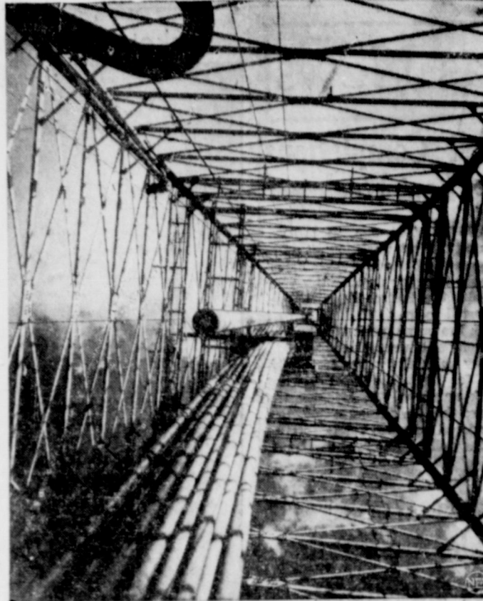
You're looking up into the world's tallest drilling rig, located in the swamps of Louisiana. This rig is the most powerful ever assembled, and is designed to drill 18,000 feet into the earth in a search for oil. That pipe you see suspended inside the rig is 135 feet long.
