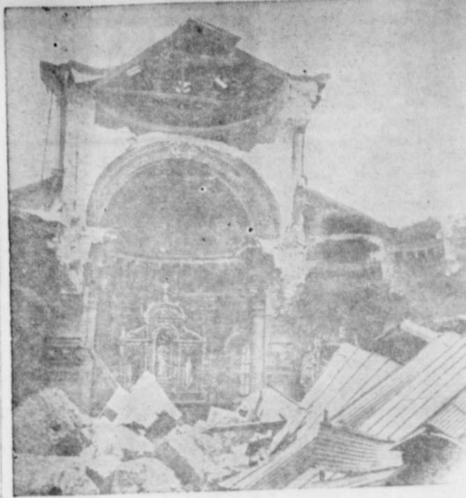
TOMB . . . Stricken by the earthquake that struck most of Ecuador, the walls of the cathedral of Ambato caved in on 60 small children who were inside the cathedral at the time of the quake.
