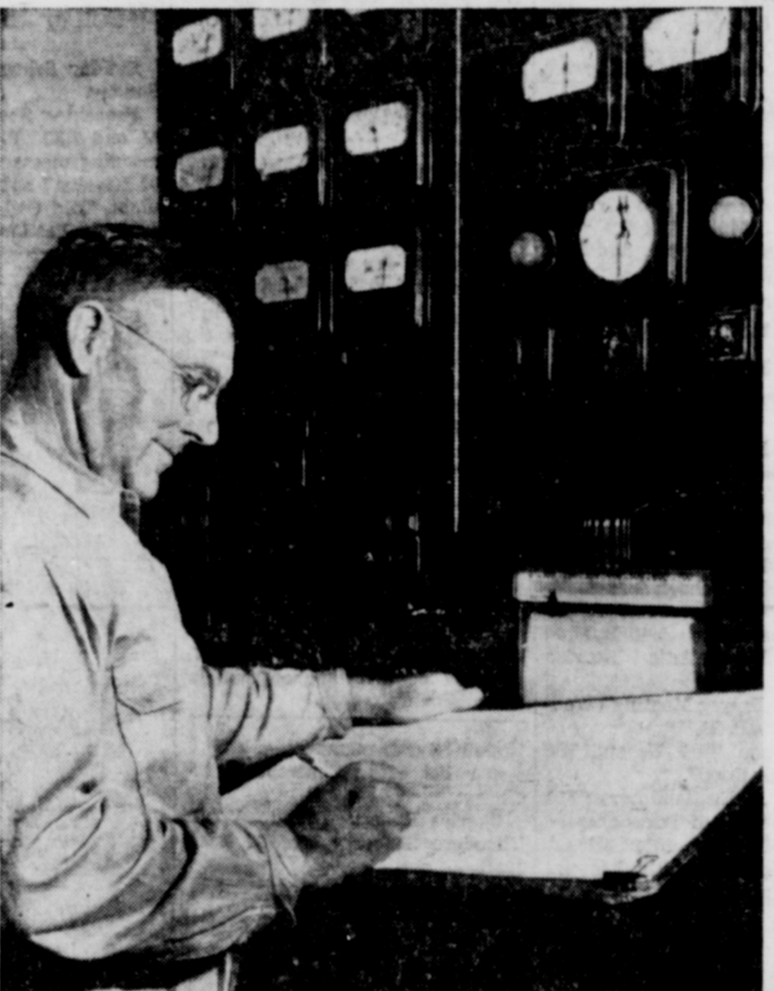
1. Close control of every process has enabled Baytown refinery to make its substantial contribution to your need for petroleum products. This is the control panel in one of Baytown's two catalytic cracking units, called "cat crackers." They enable Baytown to get more finished petroleum products from crude oil processed at the refinery.
