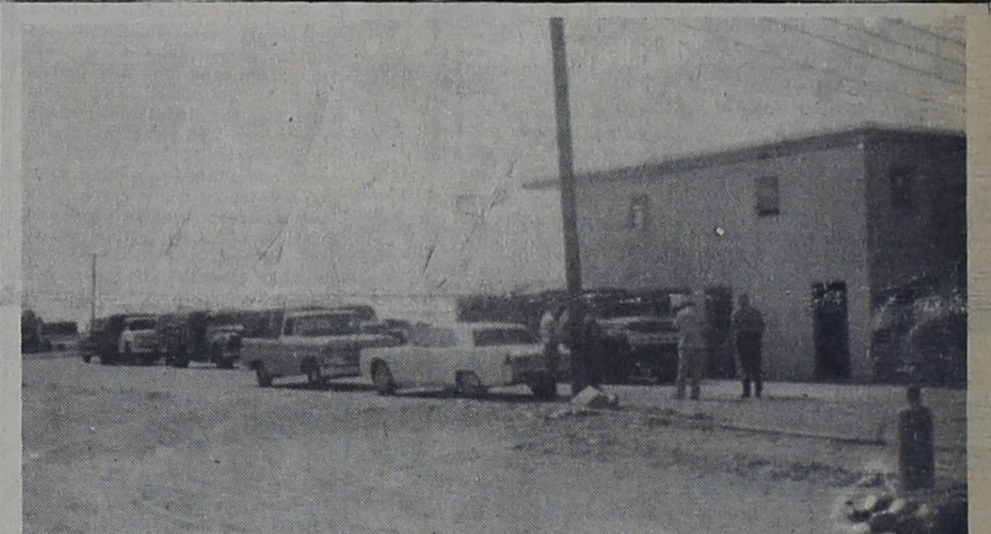
ELEVATOR OPENING--This line of trucks, loaded with wheat, were waiting for official opening of Sherry - Anderson Lazbuddie Elevator June 15. Henry Ivy delivered first load of grain to the new firm. His truck is shown parked on the scales.
