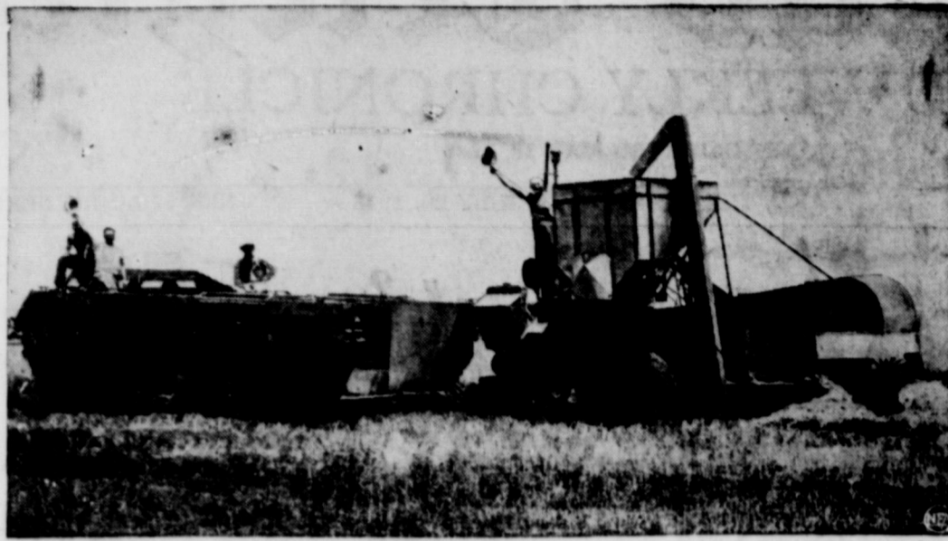
Billy Koelsch, St. John, Kan., wheat farmer, hitched his combine to a war surplus landing barge when heavy rains made his fields too muddy for ordinary tractors. Koelsch's ingenuity saved his wheat crop, which yielded about 30 bushels to the acre. With regular equipment, he would have had to wait another week before he could harvest.
