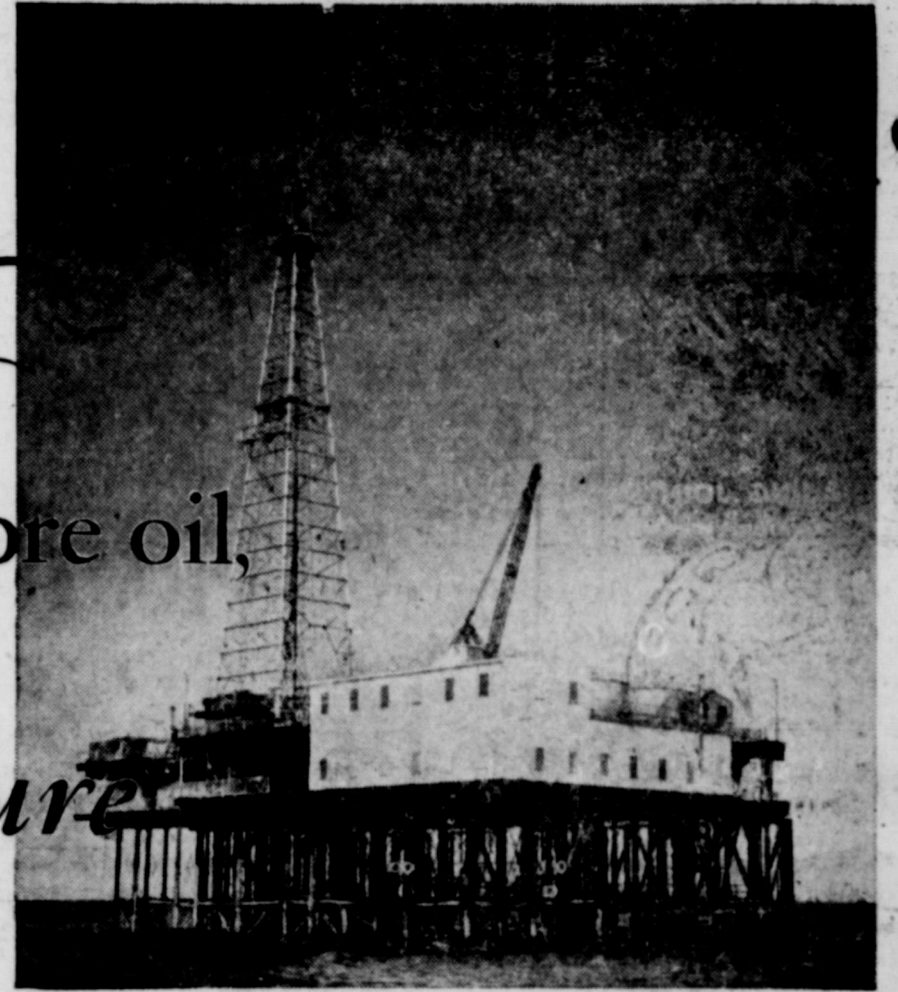
Designing and building the equivalent of a 10-story structure in the open sea called for all the ingenuity and skill of the country's best engineers. Utilizing carefully controlled directional drilling, as many as seven oil wells can be drilled from this structure.
