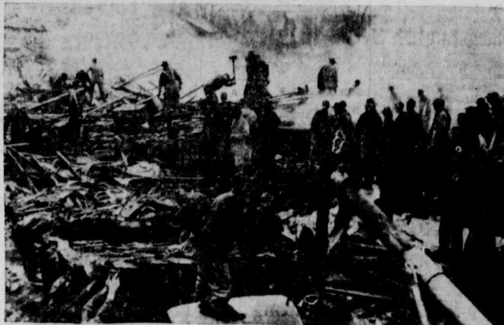
A gas-filled warehouse virtually disintegrated at Pochontas, Arkansas, in a shattering explosion which killed a Negro laborer, injured three other persons and left part of the shaken business district in flaming ruins. Body of the laborer was found just under where the rescue worker has ax poised, center background. (NEA Telephoto).
