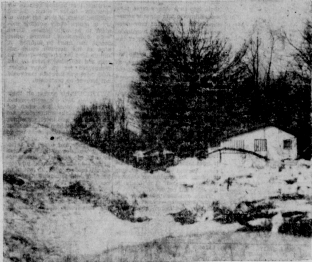
Summer homes along the Canadian shore of Lake Erie are being threatened by tons of ice, slowly advancing on the beach areas. These homes, at Erie Beach in the province of Ontario, are in the path of the oncoming ice mass, which has uprooted trees and crushed everything in its way. (NEA Telephoto).
