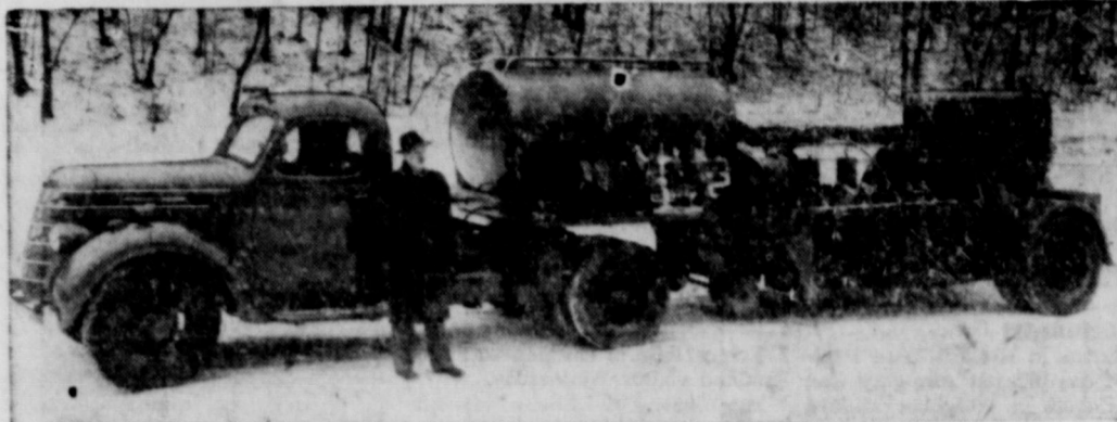
Inventor John H. Adler, of Pittsburgh, Pa., displays his "Kilroy"—a mobile filling station, which was named for the legendary war-born hero who went everywhere. Designed for service to heavy construction machinery, the station can also be used to service large aircraft and as a means of pre-construction machinery. The 21-foot trailer houses a 700-gallon fuel tank, testing sites for permanent service stations. The 21-foot trailer houses a 700-gallon fuel tank, water tank, two batteries of nine hose reels and all types of oils and lubricants.
