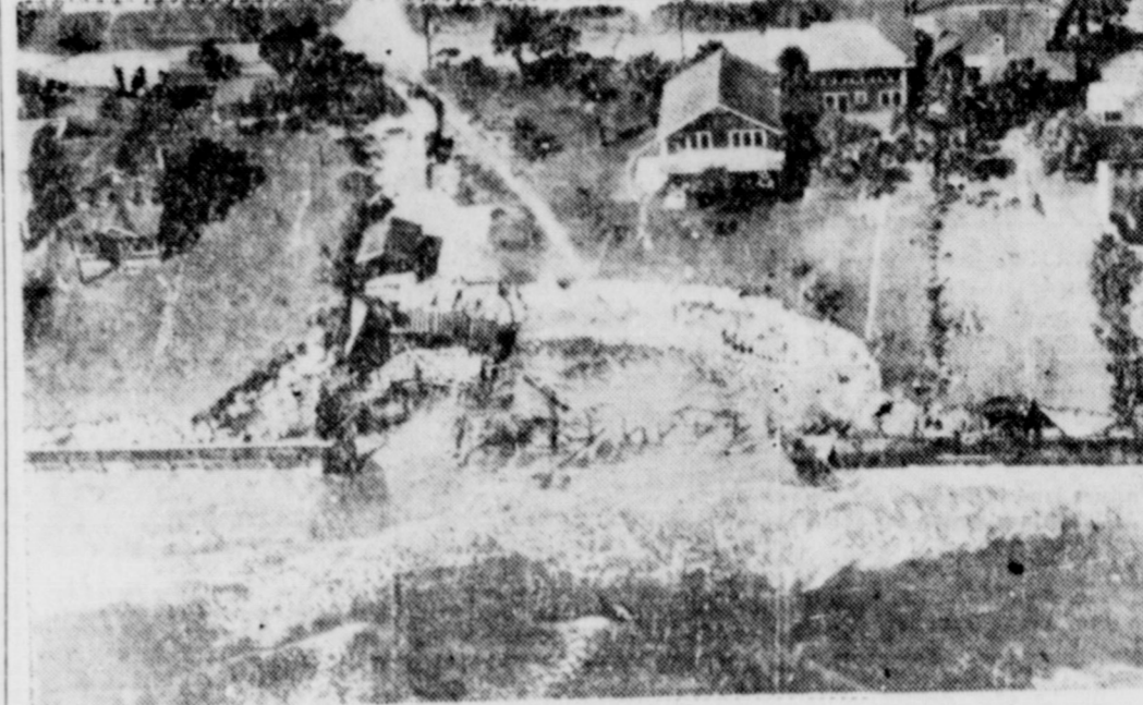
This U. S. Navy photograph, taken at Jacksonville, Florida, shows how high tides at the beach washed away part of the retaining wall and undermined a house which collapsed into the sea. (NEA Telephoto).
