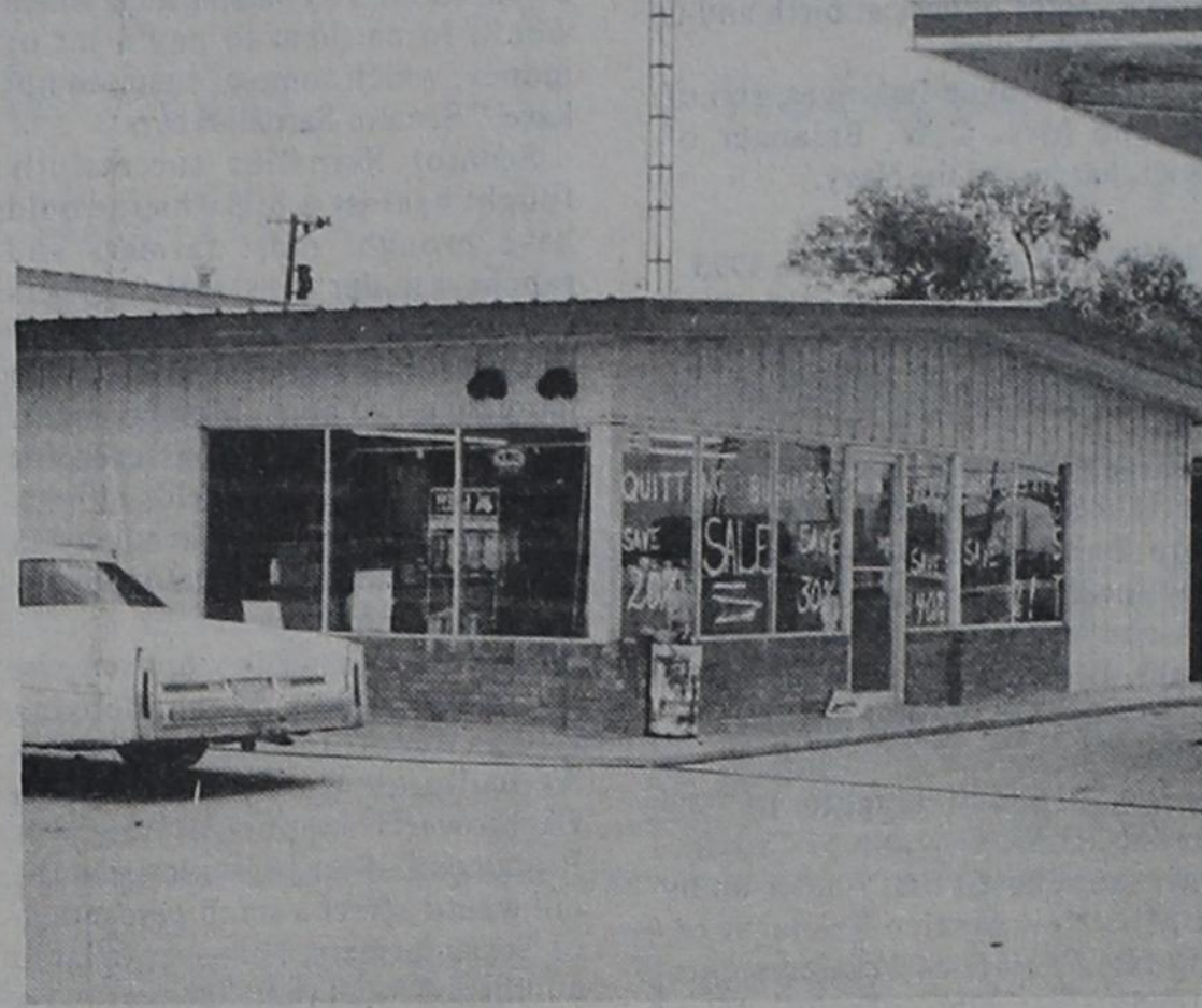
CLOSING UP.... When the Bovina Wheat Growers' fuel station closes on Friday, June 10, it will end 55 years that the company has served the farmers of the Bovina area. High interest, low farm prices and poor crops have taken their toll on the business.
