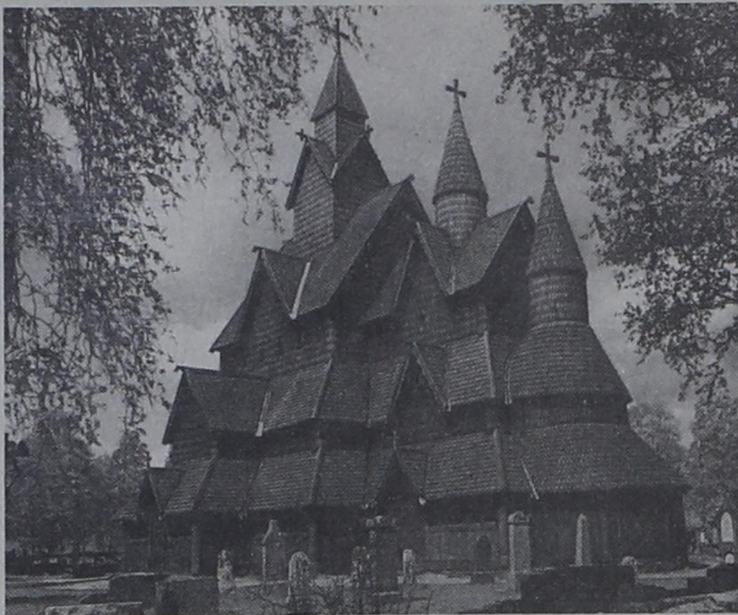
NORWAY'S LARGEST stave church, seen on tour recently by Gene and Edna Scott, as they toured eight countries. This church is dated 1147-1250 and regular church services are still conducted there. The wood is grooved and notched and boards were placed vertically. There are no nails in the structure.
