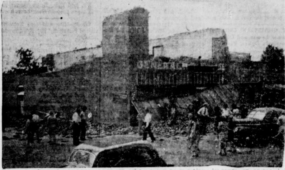
Lightning, rain and windstorms, reaching tornado proportions in some areas are doing widespread damage to crops and property in widely scattered areas throughout Texas as shown in the picture after a tornado hit Stoneburg, Texas, last week end. The two story building, above was reduced to a pile of rubble as were the two smaller buildings seen at right. (NEA Telephoto.)
