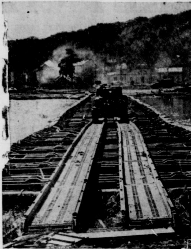
FIRST TANK rolls over a newly constructed pontoon bridge across Seine river. U. S. Army engineers built the bridge to replace one destroyed in battle. United States Signal Corps photo. (International)
