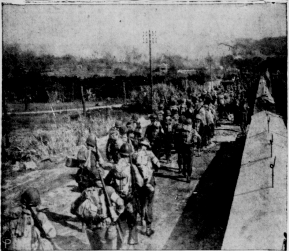
MOVING INLAND in southern France, American invaders pass the eight-foot steel and concrete wall running the length of the beach which was intended to stop such an invasion assault. A great hole blasted in the wall by assault engineers can be seen in the center of picture. (International)
