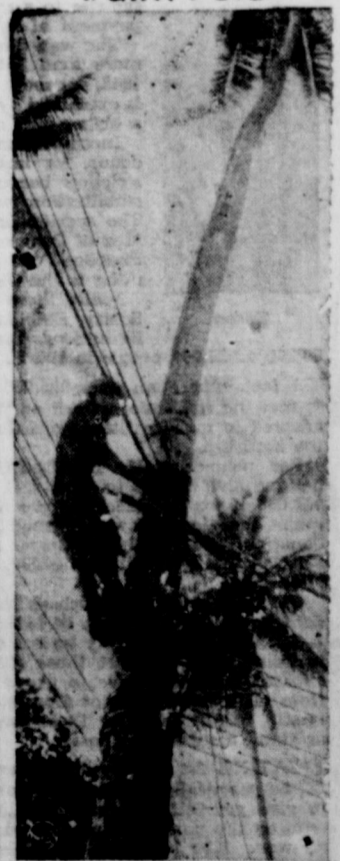
Coconut palms in New Guinea make convenient telephone poles for Army signal corps troops. Sgt. Nelson Waterbury of Ypsilanti, Mich., is the lineman hooking up communication wires near Buna. (Passed by censor.)
